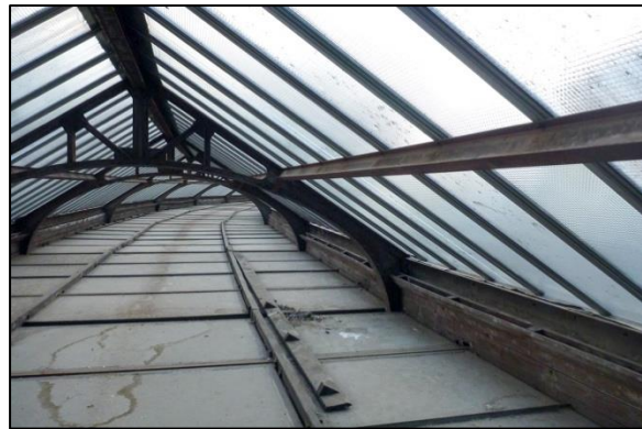
Fig. 42b: The steel and glass structure in the roof.
