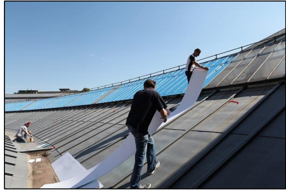
Fig 42d: Installing the forex panels on the glass structure of the Historic Gallery.
