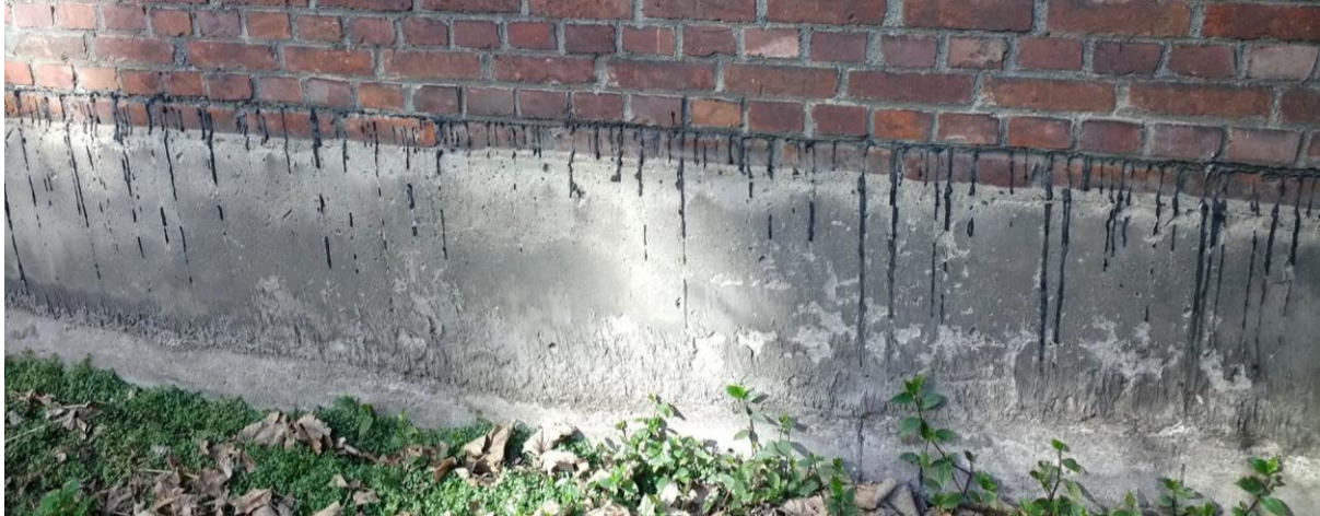
Figure 3: an example of an old (successful) attempt to avoid rising damp in a wall. The layer of tar is still efficient nowadays. Clearly the layer of tar was not applied in a very careful way, but this does not affect its efficiency.
