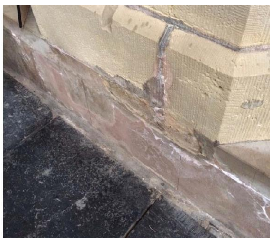
Figure 45: Efflorescence and stone damage at the base of columns. Right: detail of fig. 3.1. Note the pink colour on the base of the column (L. Miedema, 11-09-2014)
