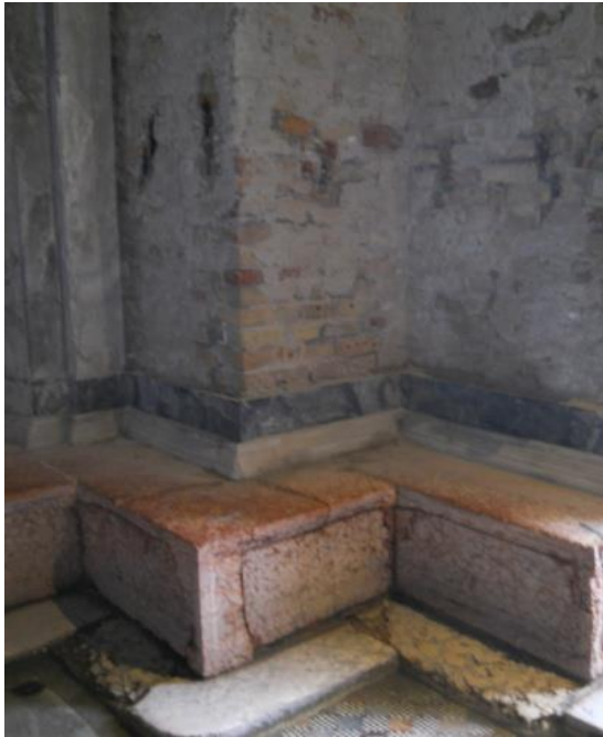
Figure 30: Pillar of the Narthex, near Zen Chapel, treated with the bars system. The bars' heads are visible on the upper part of the masonry
