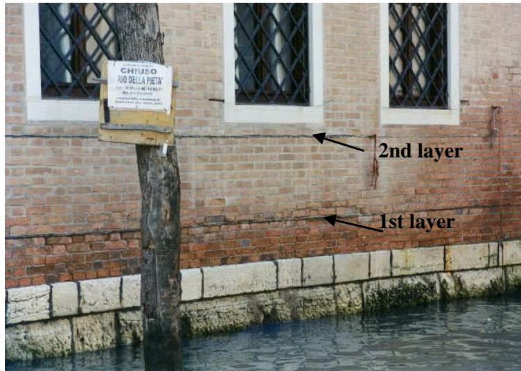
Figure 7: Presence of mechanical interruption (2 layers) in a building in Venice
