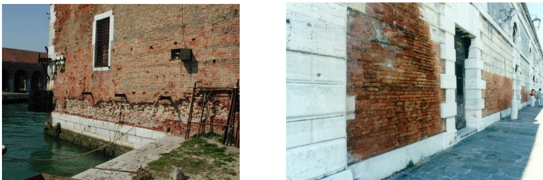
Figure 5: Alberaria Tower (Venice) and Salt emporium (Venice): horizontal courses of Istria stone blocks were used at the base of the walls to limit the capillary rise of water.
