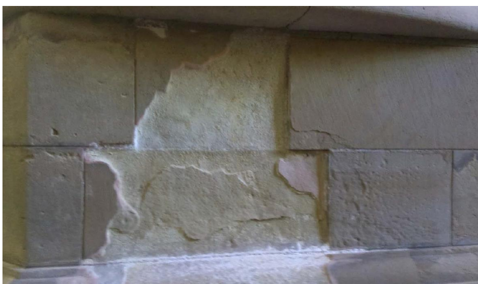
Figure 49: Scaling of stone (B. Lubelli, 09-10-2014)
