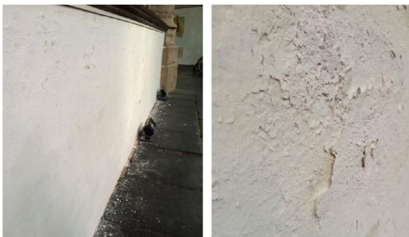
Figure 48: Damage to plaster as a result of efflorescence. Right: Detail showing damage to plaster and paint (L. Miedema, 11-09-2014)
