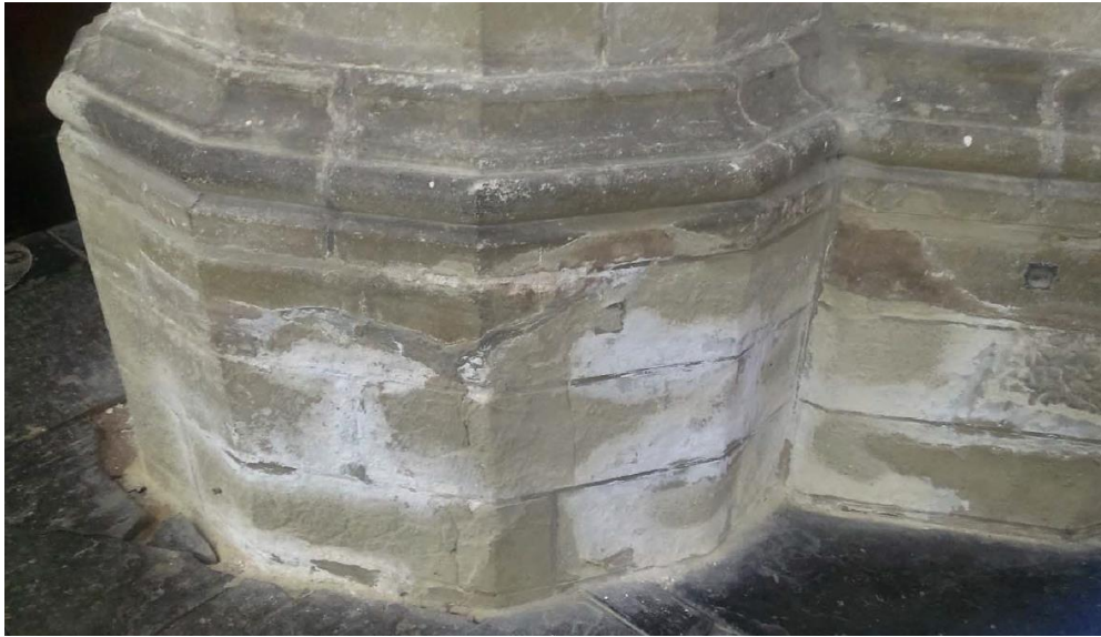
Figure 50: Efflorescence and scaling of stone (B. Lubelli, 09-10-2014)
