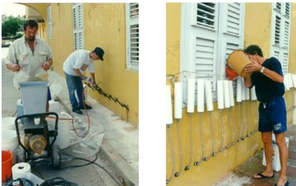
Figure 9: Treatment of a wall using pressure (injection) (on the left) and using only hydrostatic forces (impregnation) (on the right)
