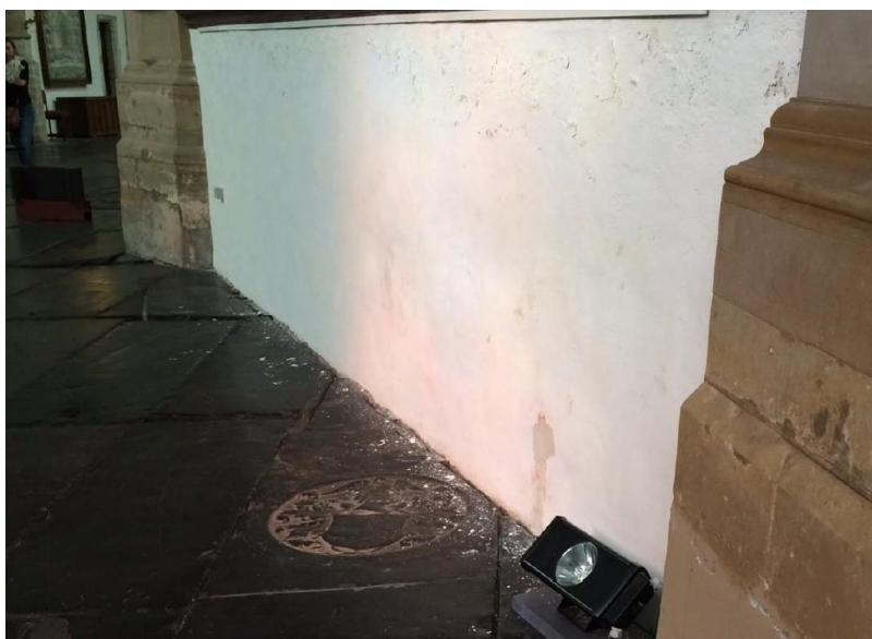
Figure 47: Damage to plaster as a result of efflorescence (L. Miedema, 11-09-2014)
