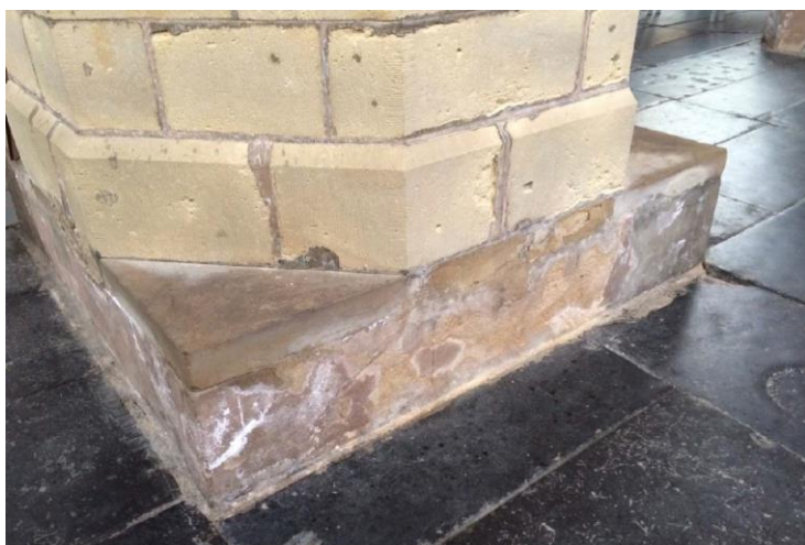
Figure 44: Efflorescence and stone damage at base of column (L. Miedema, 11-09-2014)
