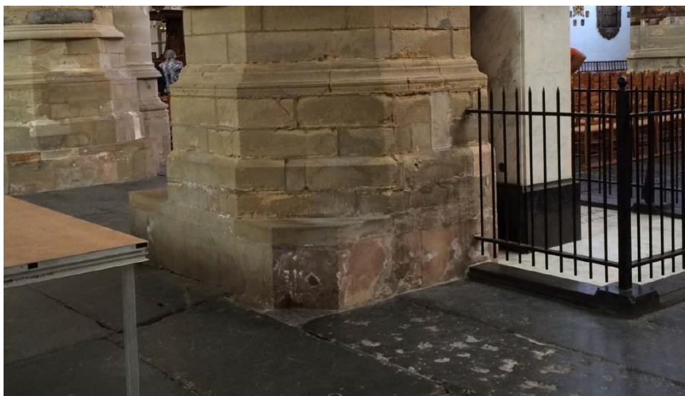
Figure 46: Efflorescence and stone damage at base of column. Damage to floor (L. Miedema, 11-09-2014)
