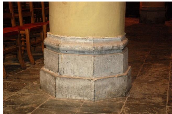
Figure 66: historic attempts to protect the building against rising damp. On the left: wall base constructed out of dense blue stone, and local sand-limestone. Notice the very thin vertical joints between the blue stones. On the right: the bases of the columns in one piece of dense blue limestone, which turns out to be a very efficient protection for the upper parts of the columns.
