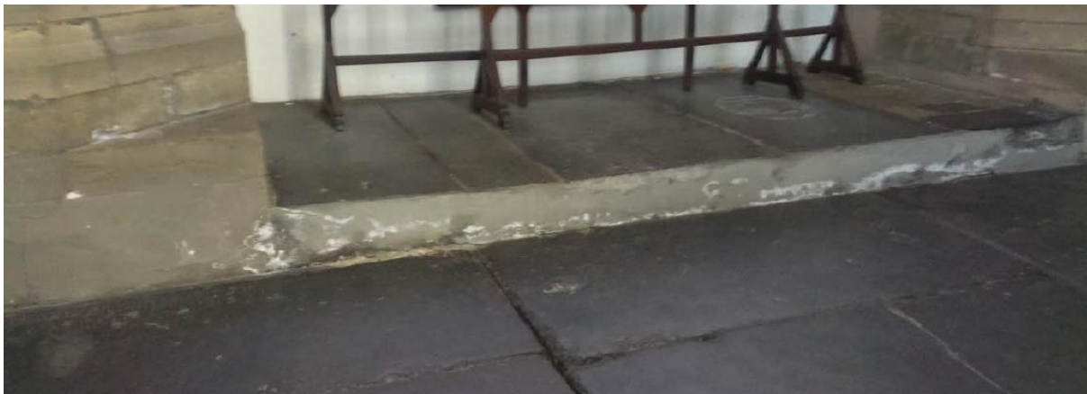
Figure 51: Efflorescence on stone (B. Lubelli, 09-10-2014)
