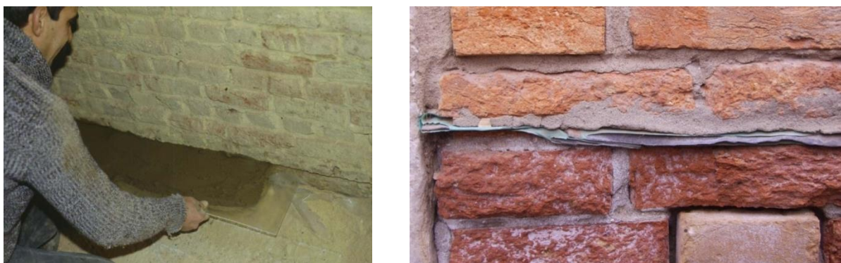
Figure 8: applications and result of a mechanical interruption
