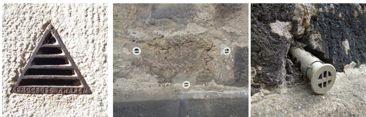
Figure 10: Different types of Knapen Siphons in a wall (Lubelli, B.)
