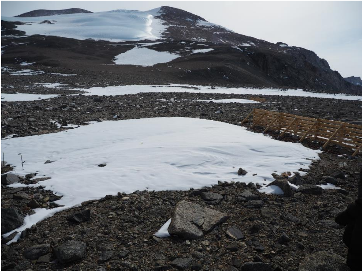
Fig. 3.2.2 Snow fences in Dry Valleys with windscoop formation behind it. The two snow fences were placed perpendicular to the wind direction, so that the snow would accumulate behind.
