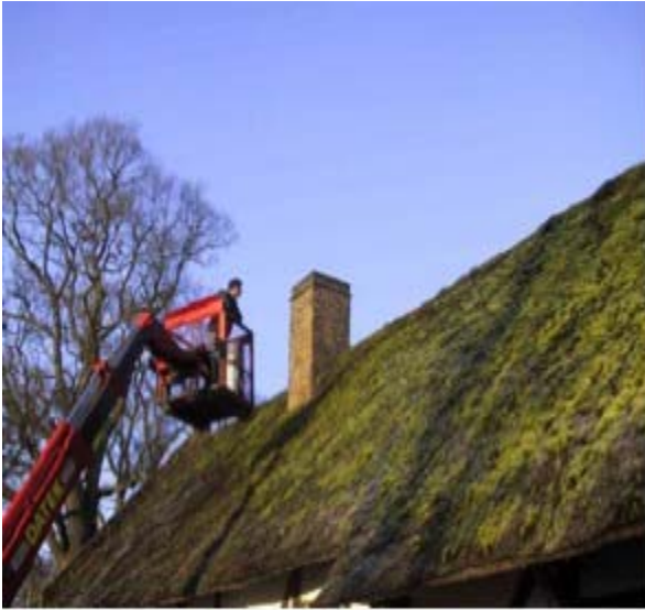
Figure 58 : Emission measurements at the chimney of one of the houses in the Bokrijk museum
