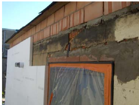
Figure 1: Outside insulation placement in Antwerp demonstration project: the roof has been insulated first, providing a roof extension for better connection with the outside insulation. 8
