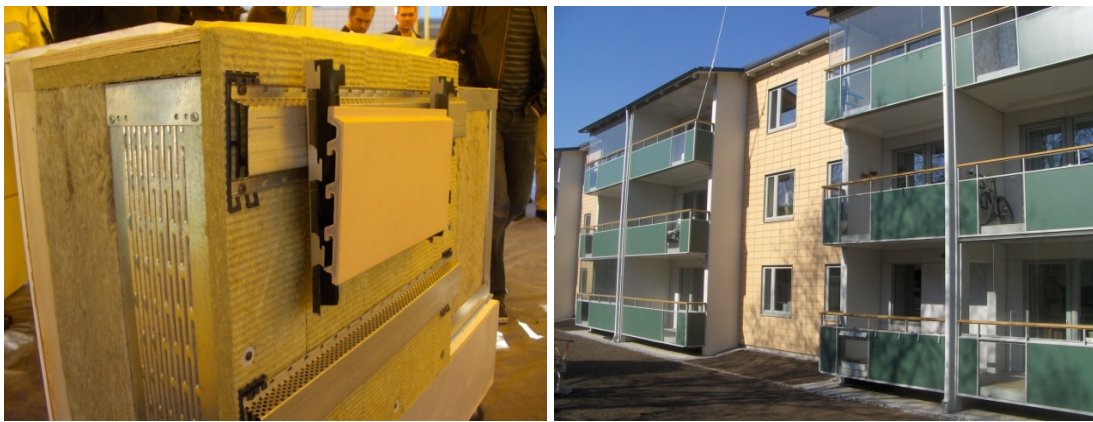
Figure 4: Prefabricated wall retrofit system used in the renovation project Brogarden, Alingsås, Sweden 10 . The outside façade was removed and replaced with a fully prefabricated new façade. Optimization of the system after experimentation with a first demo project allowed for further cost reduction (IEA SHC Task 37).
