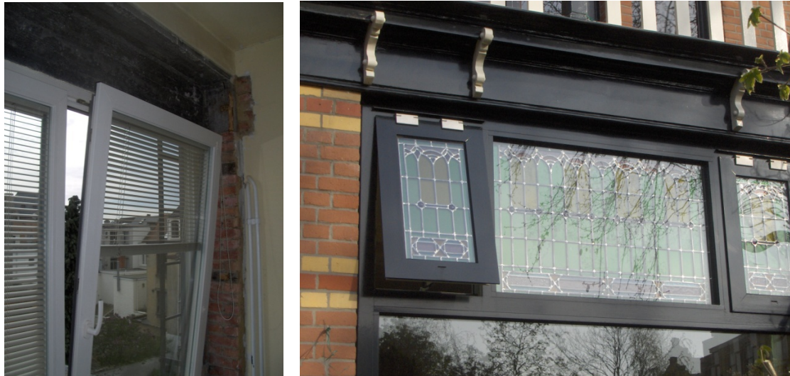
Figure 11: Left: Triple glazing with integrated solar shading and winter/ summer ventilation mode. (Renovation project Victor Driessensstraat, Antwerpen); Right: Renovation of glass-in-lead windows in a protected housing area in Rijswijk, the Netherlands: the glass-in-lead is carefully removed by the specialized manufacturer and integrated in a new frame. 23
