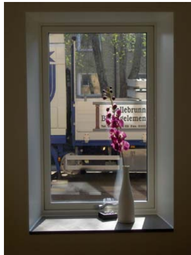
Figure 10: Inclined wall sidings after retrofit allow better daylight intrusion from small windows after retrofit (renovation project Brogarden, Alingsas, Sweden). 21
