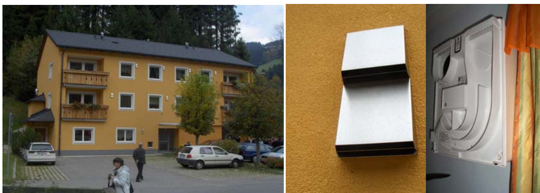
Figure 13: Decentral room-based ventilation solution with heat recovery in a visited demonstration project in Gasen, Austria.
