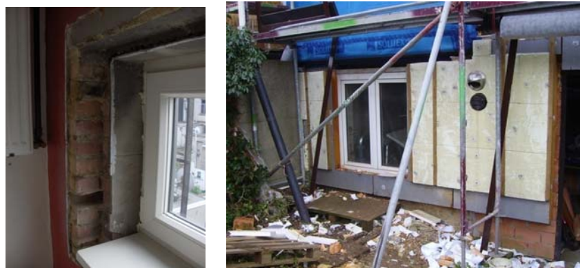
Figure 8: Left: Minor impact on interior finishing with the replacement of a window and window tablets. (Renovation project Antwerpen). Right: Putting windows and insulation into place usually implies scaffolding and workers carrying materials through the house: this has an important impact on the garden (Renovation project Deurne). 18
