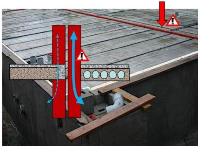
***Figure 30: Hollow core slabs and concrete slabs must bear upon all supporting walls which continue through to other storeys. This may involve supporting on four sides. If this is not assured, significant sound transmission between storeys may occur through the wall.***
