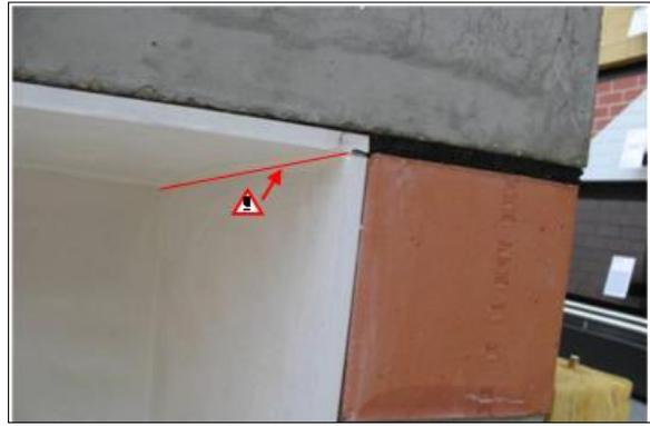
**Figure 25:** Structural building concept 5: using a cutter, cut the plastering at the joint between the slab and the wall through into the resilient layer, in order for vibration coupling to be avoided here as well.
