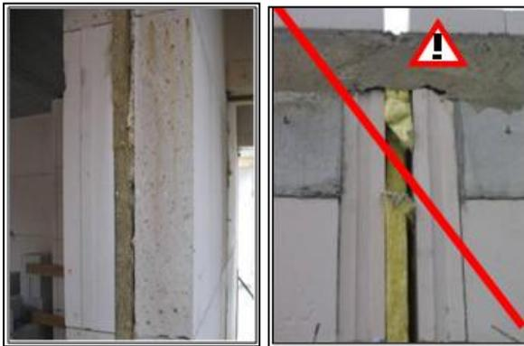
**Figure 26:** Very high sound insulation levels ( $R_w > 65$  dB) can be obtained by means of a double wall of sand-lime brick ( $m'' > 250$  kg/m<sup>2</sup>) provided no rigid contact exists between the party wall leaves. Serious errors may however be made at the level of the floor supports. With coupling as shown by this figure, the sound insulation can easily drop by 10 dB or more.
