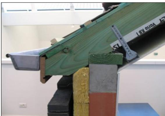
**Figure 38: Photograph of installation of a decoupled suspended ceiling and transition to outer wall**
