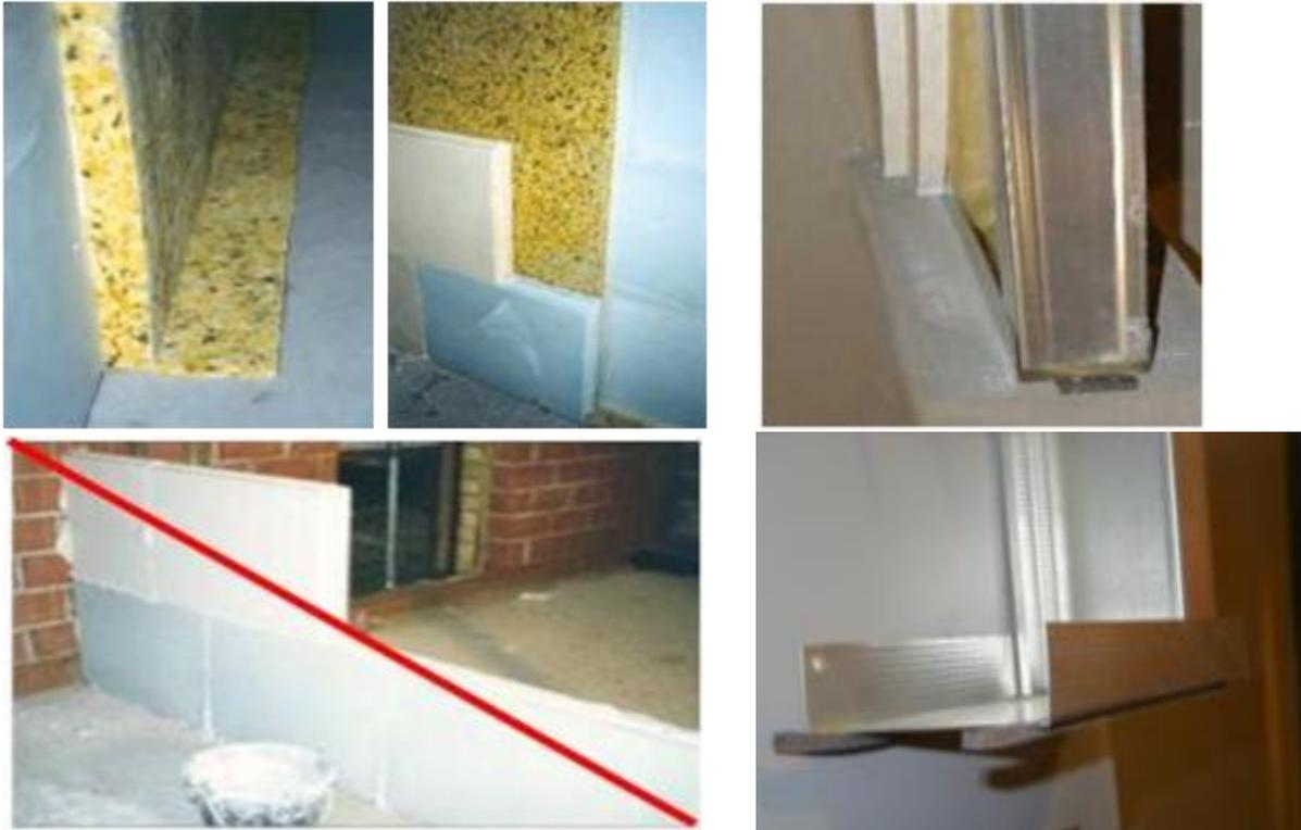
**Figure 42: Gypsum blocks must also be decoupled resiliently from the floor slab by a suitable resilient strip. At the periphery, a permanently resilient joint is employed at the transition for the surface finishing.**
