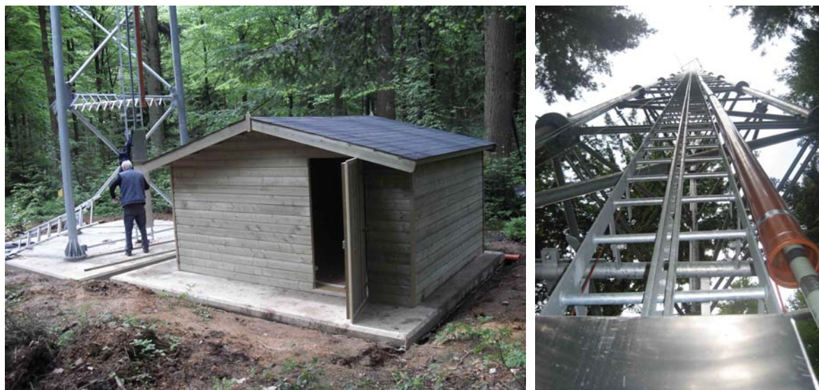
Figure 28: Left: the new shelter and the bottom of the new tower. Right: the new tower equipped with tubing for BVOC sampling at the top of the tower (orange tube).
