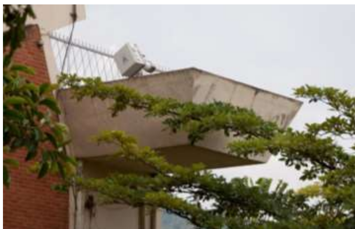
Figure 38: MAX-DOAS instrument installed on the roof of the Physics Department building of the University of Burundi, in Bujumbura (3°S, 30°E).
