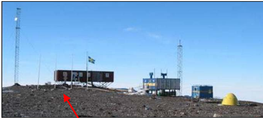
Station on rock (Wasa)
