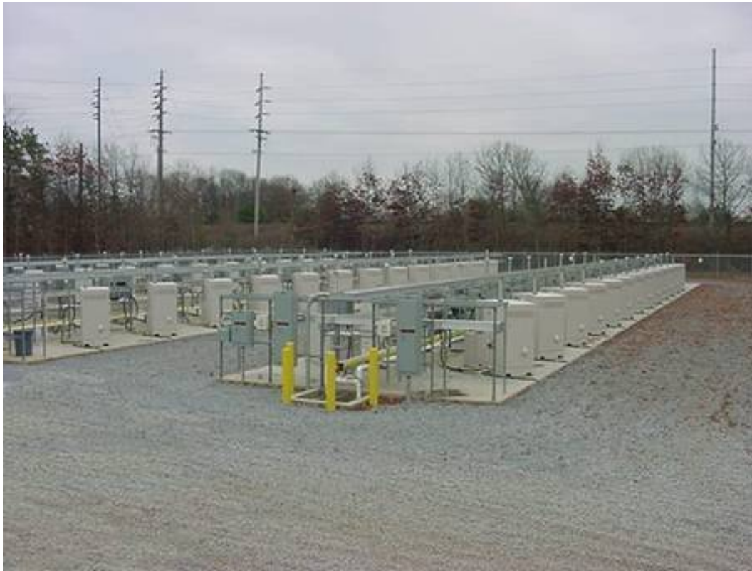
Figure 2-12: 75 fuel cell units acting as an electricity plant at Long Island Power Authority.
