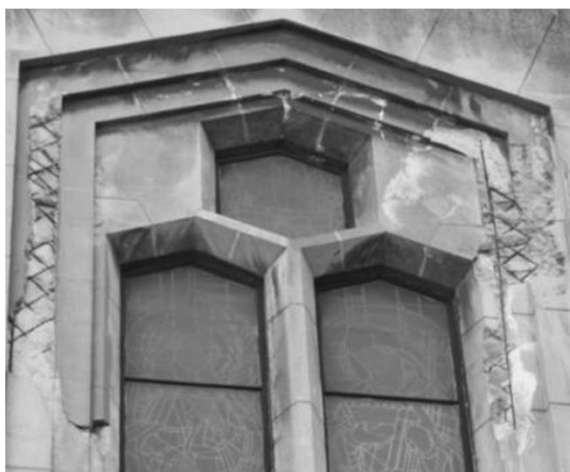
Figure 33: Spallings around the North West bay of the choir, Saint-Vincent Church
