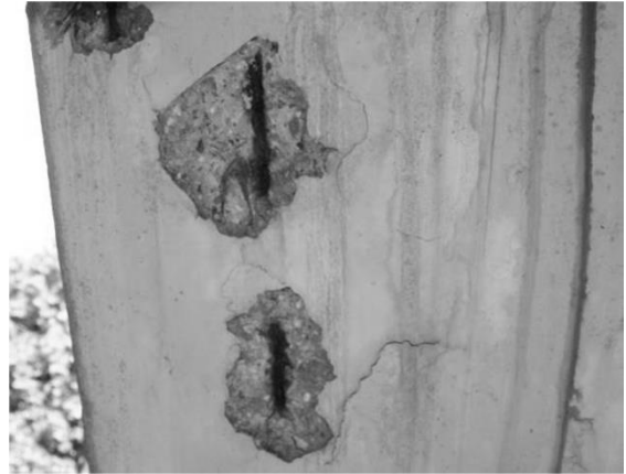
Figure 11: apparent reinforcement and rust marks on the bottom side of the stairs leading to Sainte Virgin Mary
