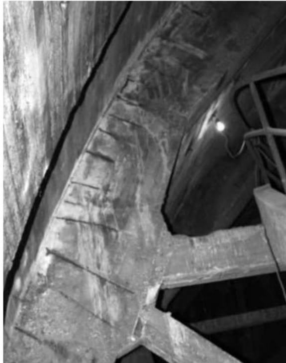
Figure 23: Reinforced concrete frame structures (between dome shells)
