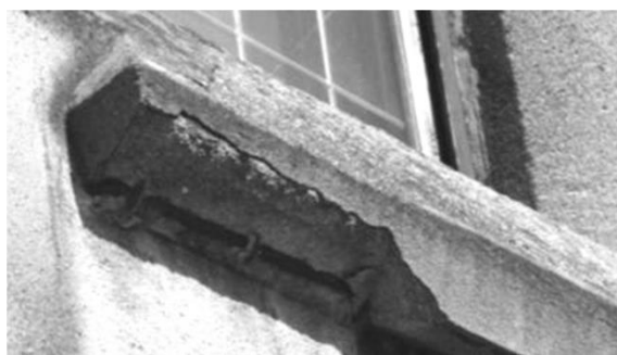
Figure 33: Spallings around the North West bay of the choir, Saint-Vincent Church
