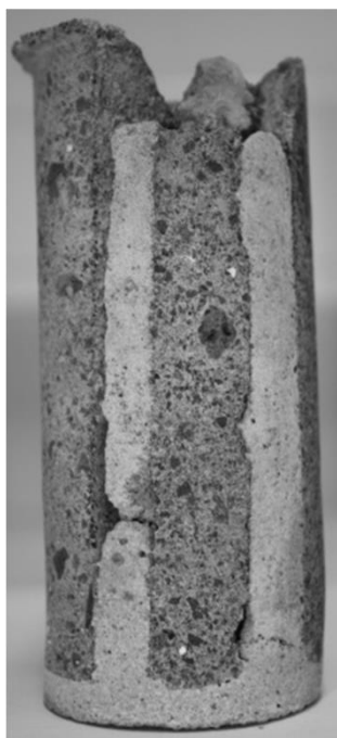
Figure 24: Sample of concrete (internal wall, Saint-Vincent church)
