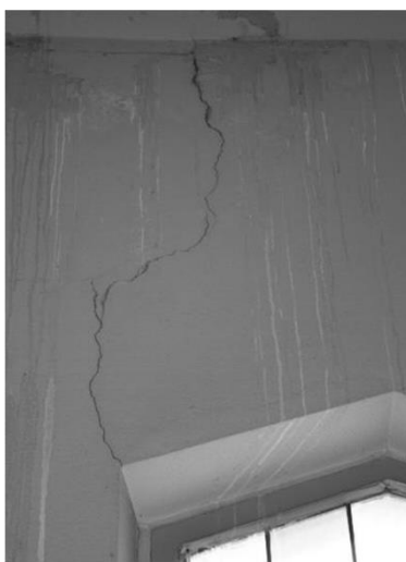
Figure 12: crack with various direction, appearing in an opening's angle (Saint Vincent's west facade)
