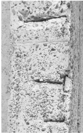
Figure 10: apparent horizontal reinforcement on a pillar (Saints Peter-and- Paul's west facade)
