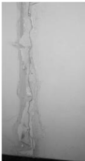
Figure 13: vertical crack in a pillar on the left of Saint Vincent's organ
