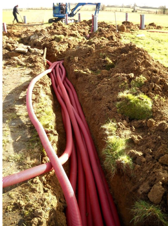
Figure 7 Excavation made for the pipes
