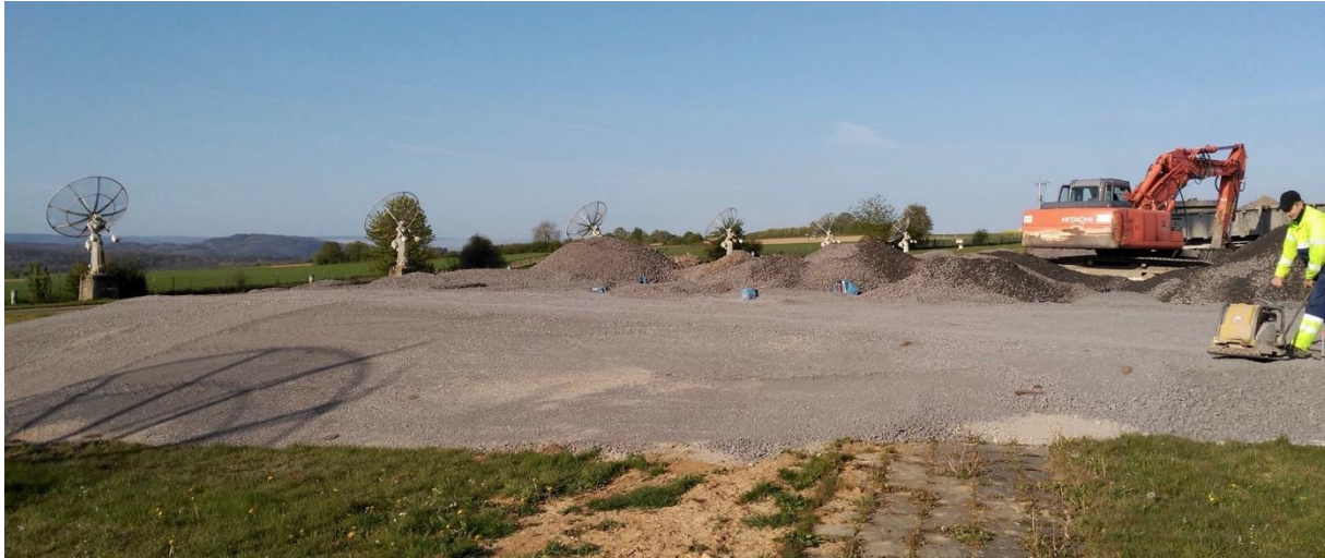
Figure 8 Construction of the foundations of SPADE
