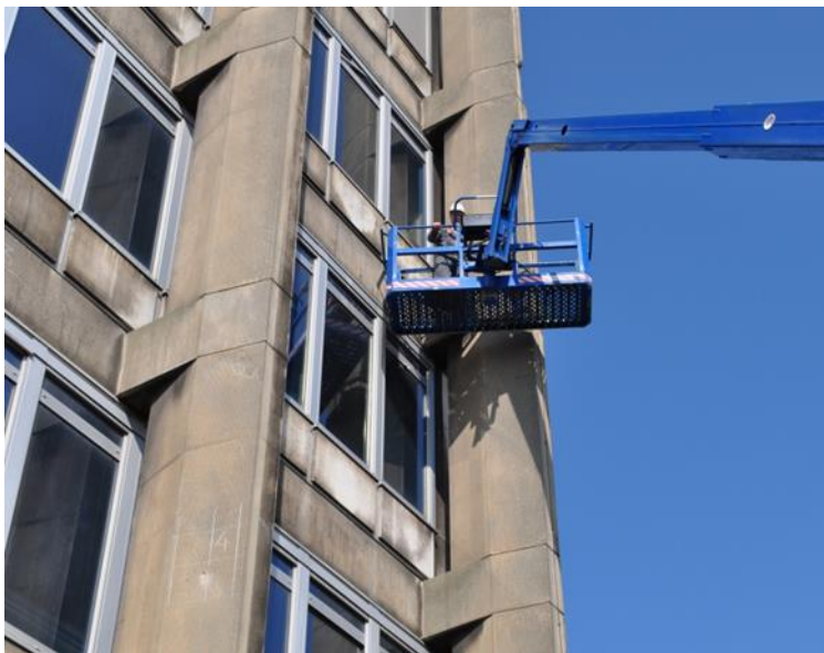
Figure 2 – Diagnosis of the police tower Oudaan in Antwerp (architect: Renaat Braem)
