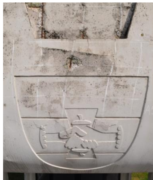
Figure 1 – Porch roof of Building M of the VUB (architect: Renaat Braem)
