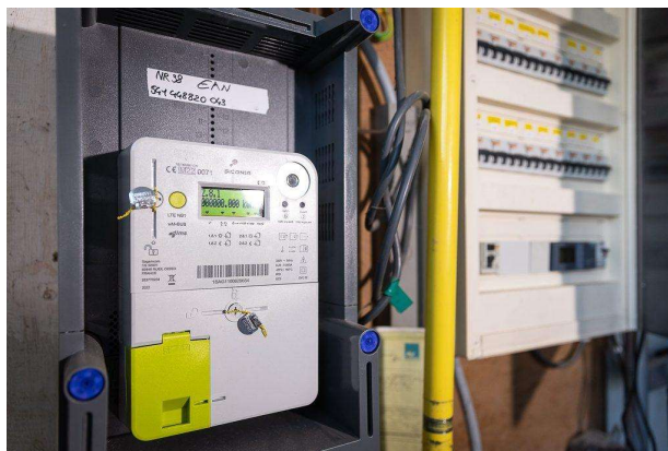
Fig. xxx: illustration of a smart meter used for billing electricity and/or gas (or water)
