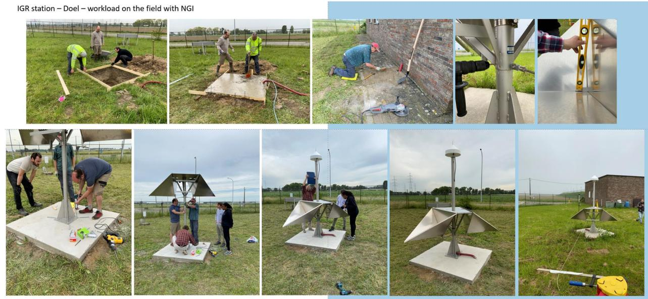
Figure 114. Manual fieldwork done in successive visits on the field in Doel allowing a sequence to fully install the antenna, to connect the electricity and install the modem with the SIM card and to install and correctly oriented the IGR antenna.
