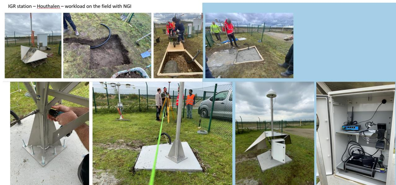
Figure 116. Pictures taken on the field during the successive phases to dig the trenches (allowing to bring the electricity cables to cabinet of the IGR station) and the square base dug for the creating the concrete basement. The cabinet containing the modem and the recorder is shown also.
