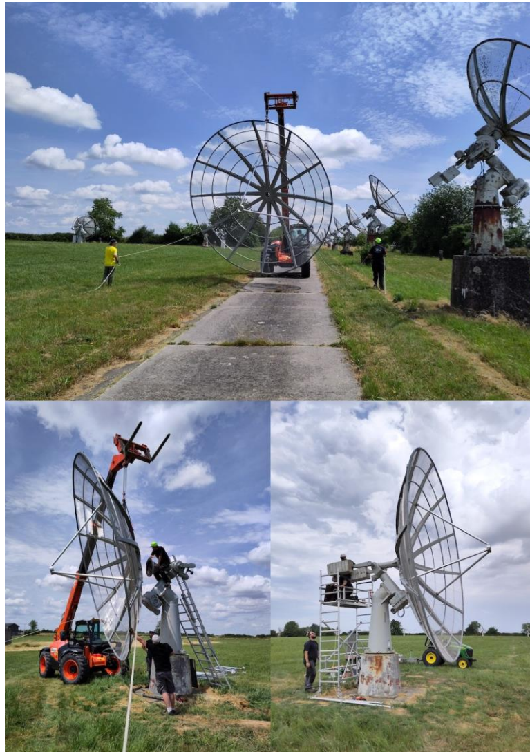
Figure 5: Top: transportation of the refurbished parabola inside the station; bottom left: the mount is reinstalled, and the parabola is being fitted to it; bottom right: fastening of the counterweights
