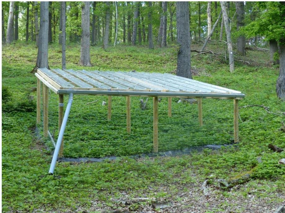
**Figure 6. Partially covered roof installed above seedlings to induce artificial drought**
