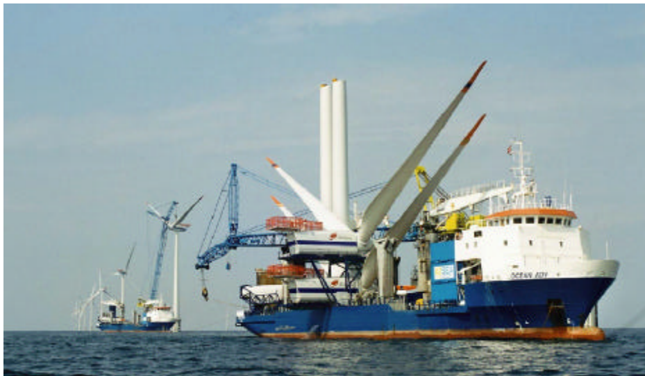
Figure 27: A2SEA vessel used for the installation of the Horns Rev wind farm in 2002 (from A2SEAwebsite).
