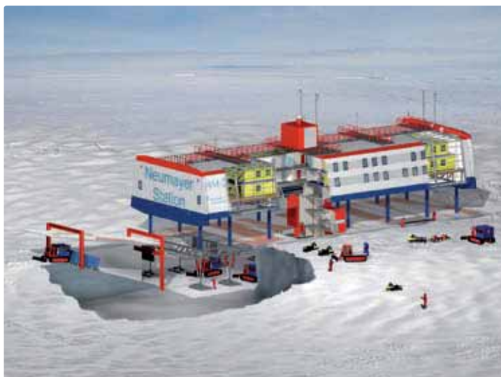
© Alfred-Wegener-Institut Germany (Neumayer Station III)
